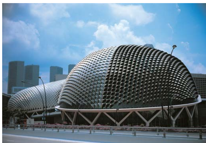
The elaborate window cladding system is a key element of the cooling system of the building - photo courtesy the Esplanade Company Ltd Photo: Eujin Goh
