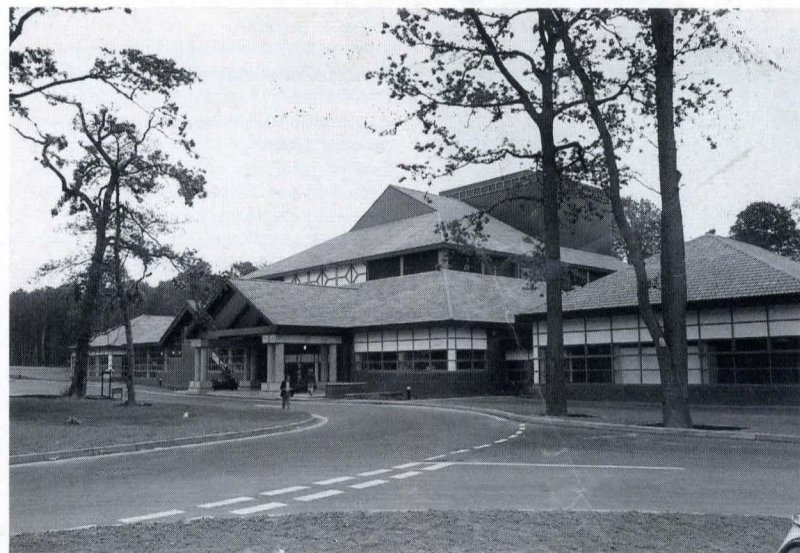
The New Hawth Theatre, Crawley. Architects Norman and Dawbarn in Association with the Crawley Borough Architect.
