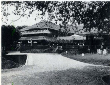
On a superb Thames side site – the brand new Caversham Hotel.
