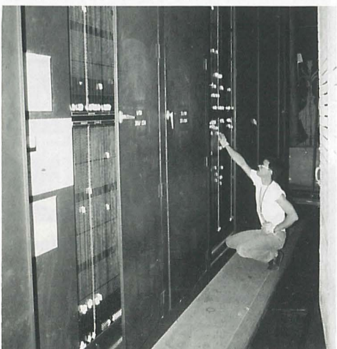
Back stage, the magnificent old Electro sliding contact patch panel. All this has come down to a key pad on current Electro systems!
