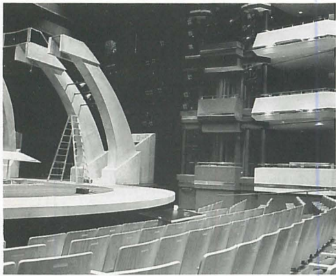
The Max Bell Theatre. The triple tier of stage boxes painted in the darker shade pivots to suit variable proscenium width on an air castors—but not while occupied! Lighting control by Electro 'Premiere'.
