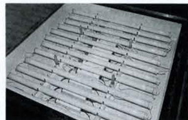
The tubes and Environ ballasts beneath one of the 'white' squares.
