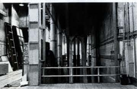
This enormous lift lowers lorries full of scenery down to stage level at the Victorian Arts Centre, Melbourne.
