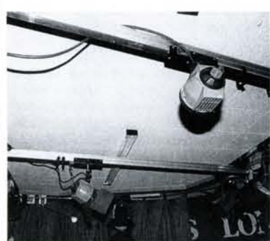
Head height at a premium! Light Rig channels installed just below the ceiling in A.B.C. News London Studio.
