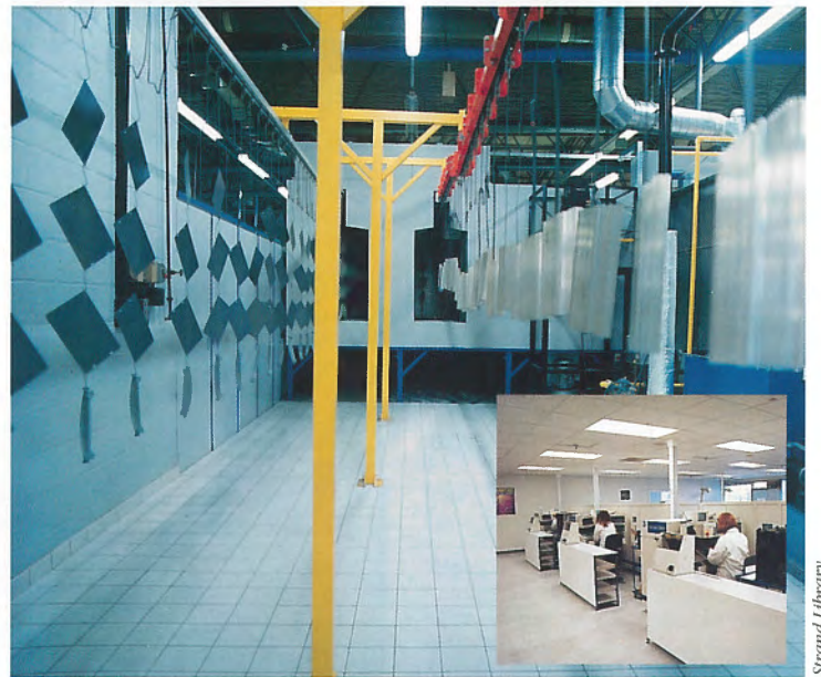
Part of the new electrostatic paint plant with the PCB facility (inset).
