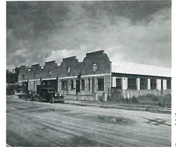
The 'new' Strand Electric factory, Power Road, Chiswick - 1932, see 80th anniversary articles.
