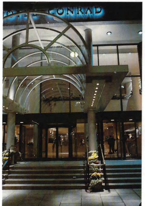
■ Hotel Conrad, Dublin: Low voltage fittings give an extra depth by uplighting the barrel vault's steel ribs and downlighting the planting on the steps.
