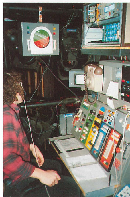
The Olivier Drum Revolve controls. The VDU on the left and electronics crate top right were added to give digital position input and greater safety. Three television screens out of picture on the right add views of understage areas to the direct view of the stage from the perch.
