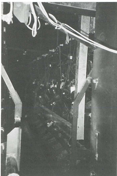
The new lighting bridge built above the Olivier stage.
