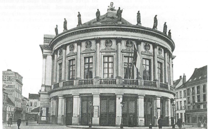
Theatre Facade (David Wilmore Collection)
