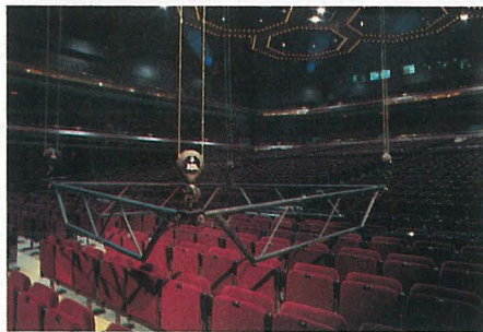
Winch spotlines can be dropped through any of the 'eggs' in the crate.
