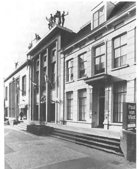
The exterior of Twentse Schouwburg. The original mixed vintage facades were retained for cost reasons but were rejuvenated with a series of life size statues of actors, singers and dancers tumbling down the facade.
