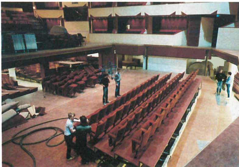
Derngate, Northampton. One of the seating waggons being brought up on the two element elevator from the basement. Other seating is stored under the stage on the left.
