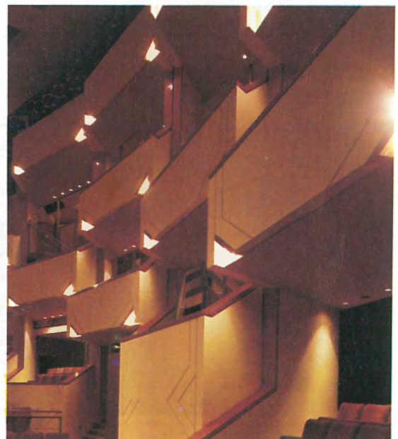
Derngate, Northampton. The two towers in the foreground contain seating at three levels and can be readily moved on air castors to give different performance formats.
