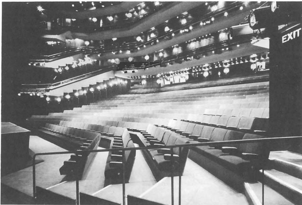
Looking across the stalls. The line of the safety curtain in front of all of the acting area is apparent and the rows of seats with a door at the end of each row except in the front five rows. The overhang of the three circles is evident – the just-in-view fourth 'circle' is the back lighting bridge, which also houses positions for the follow spots.
