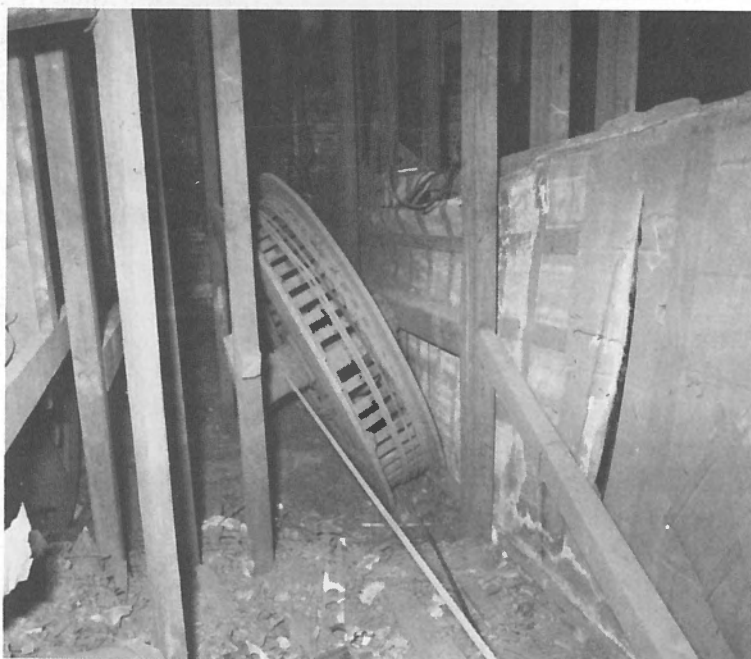
The No. 2 Bridge drum and shaft in collapsed state (photo Tyne & Wear County Council)
