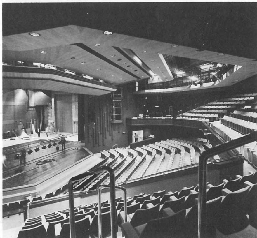
The auditorium with ceiling lowered to exclude the gallery. (Photographs by Martin Charles)
