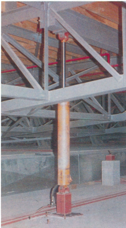
One of the hydraulic rams which adjust the rake of the auditorium floor.
