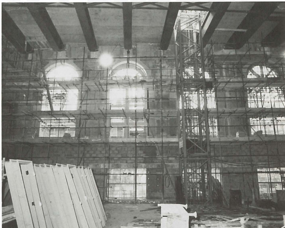
Without unduly altering the scale, windows are slightly enlarged to improve the light in the modern interior. (photos Richard Belsham)
