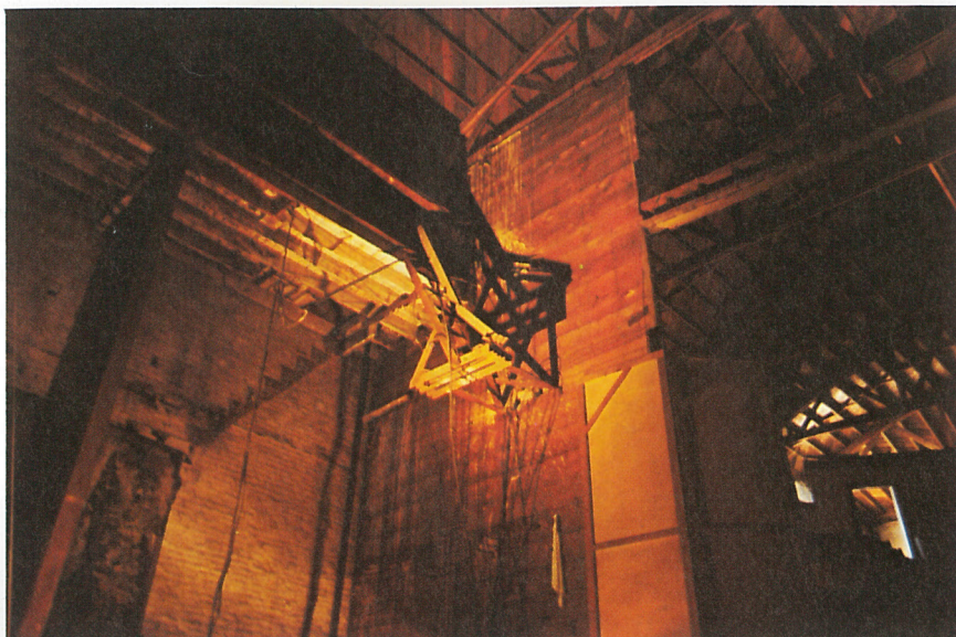
A Groove! In situ! As late as 1896! To those who know what they are a rare, rare sighting. Scene changing system pre-dating flying – there are whole libraries on the subject. No space for further explanations. (Photo Iain Mackintosh)
