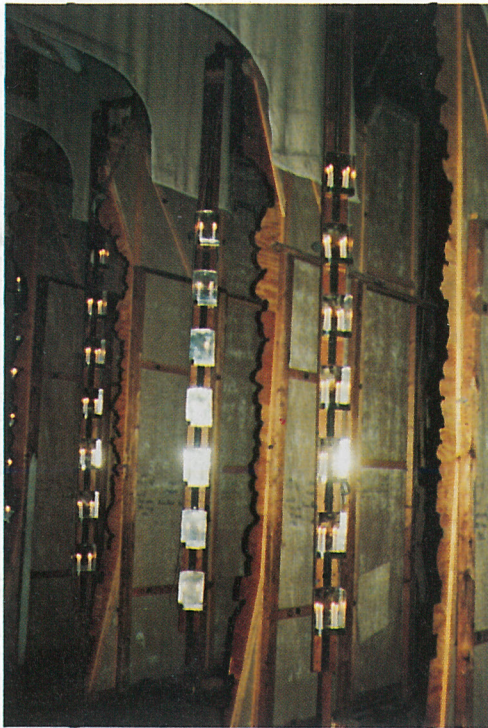
The original wing lighting poles have recreated reflectors with Cima electric candles.
