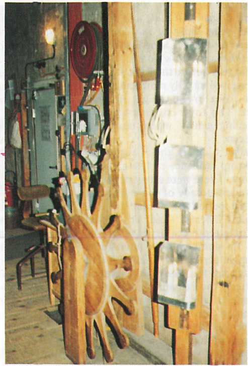
The master dimming wheel by which all the wing candle poles can be rotated towards or away from the stage.
