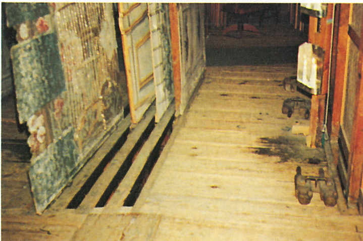
In the stage floor are the scenery grooves through which scenery flats are changed by transporting them on and off stage on understage carriages (Note candles in 18th cent shinbuster position)
