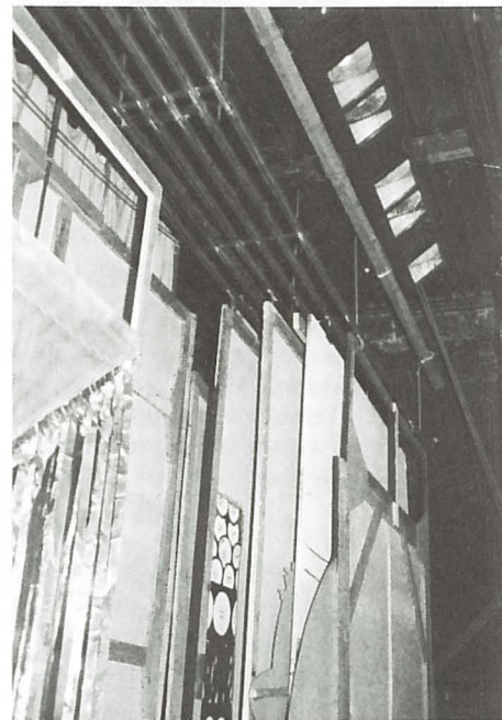
Henderson tracks for scenery suspension solved the problem of storing and handling scenery with a small performance crew.
