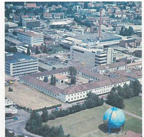
The NIETHAMMER Plant
