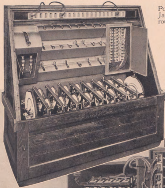
Portable Dimmer equipment made especially for the spectacular show, "Mecca," using Vitrohm round plates and Ward Leonard control levers on the switchboard.
