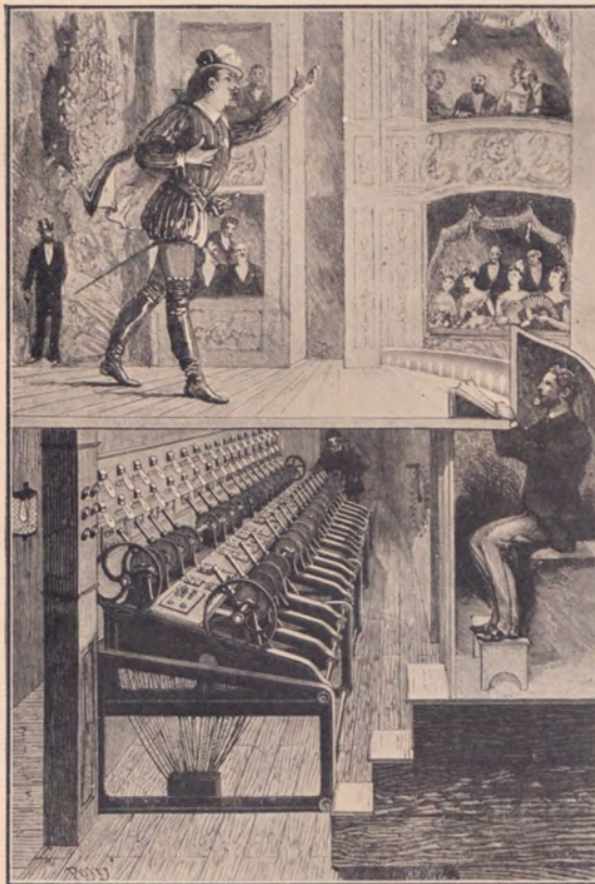
Figure 23—The electric lighting and control system used in the Paris Opera and described in L'Illustration , June, 1887. The insert shows the comparison between electric and gas batten lights and wing lights. The dimmers are extremely interesting. It will be noted that the rheostats are mounted below the floor, and the leads brought up to contact buttons, connection to which is manipulated by means of lever arms. These lever arms can be adjusted independently or locked to a master shaft which is operated from the end by hand.
