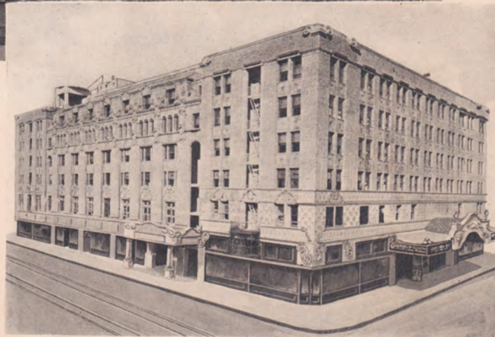
Grauman's Metropolitan Theatre, Los Angeles, designated on the coast as the "Show House of the World." Holmes and Sanborn, Consulting Engineers.
