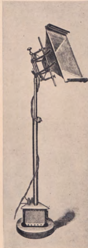
Figure 35—Spot light using an electric arc and providing for color screens, representing practice in 1898. From The Electrical World , May 1898.
