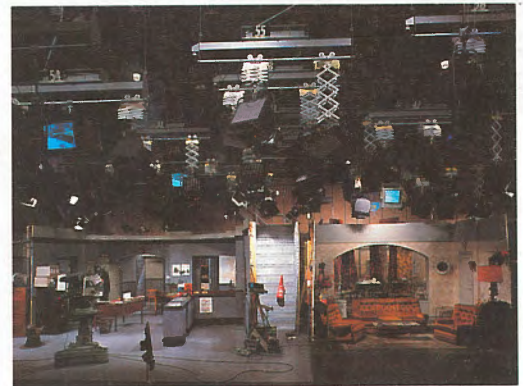
▲ BBC Wales, Cardiff, Studio C1. The first TV studio in the U.K. to use Strand's MMS memory lighting system. Equipped with Quartzcolor luminaires.
