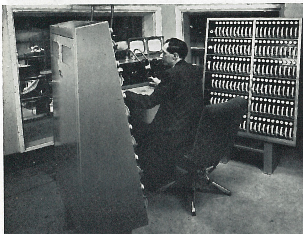
240 channel memory and preset control desk Strand System C. Four of these are in ATV Elstree Studios.
