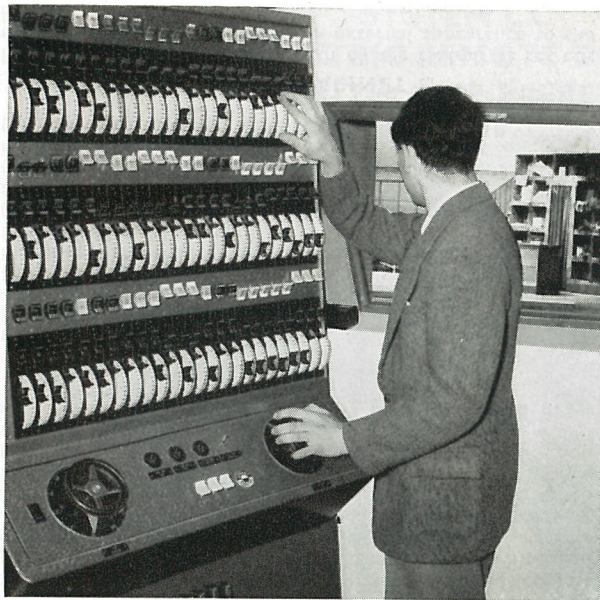
Adelaide University, Australia. Strand all-electric Saturable Reactor remote control.
