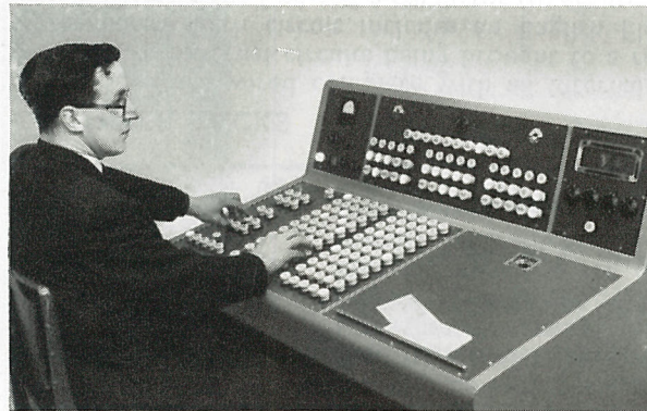
Strand system KTV. (patent applied for). The first dimmer system with fully automatic plotting of lighting and switch-board controls in the world (April, 1959).
