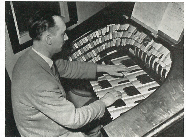
Drury Lane Theatre. Earlier form of remote control—Strand Light Console, 216 dimmers. (Photo by courtesy. "Radio Times")
