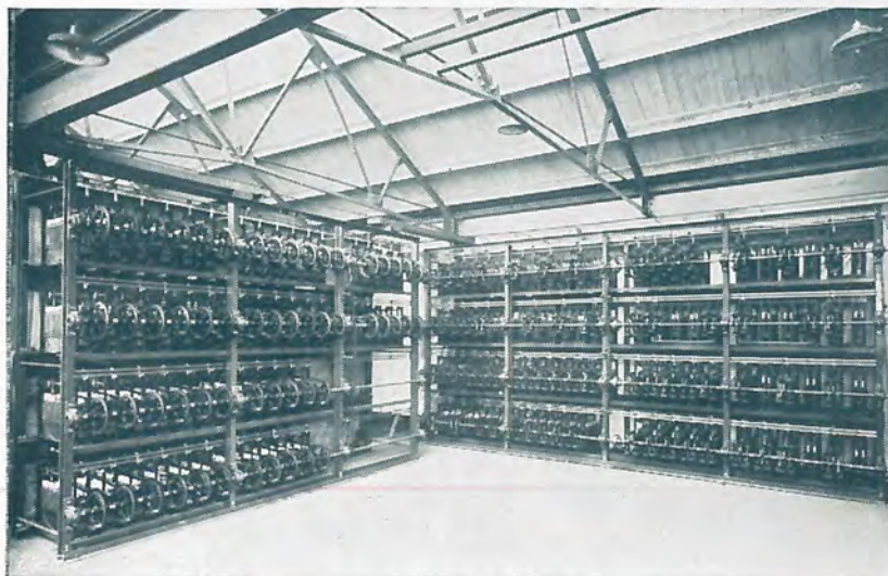
Covent Garden Opera House Dimmer Bank
