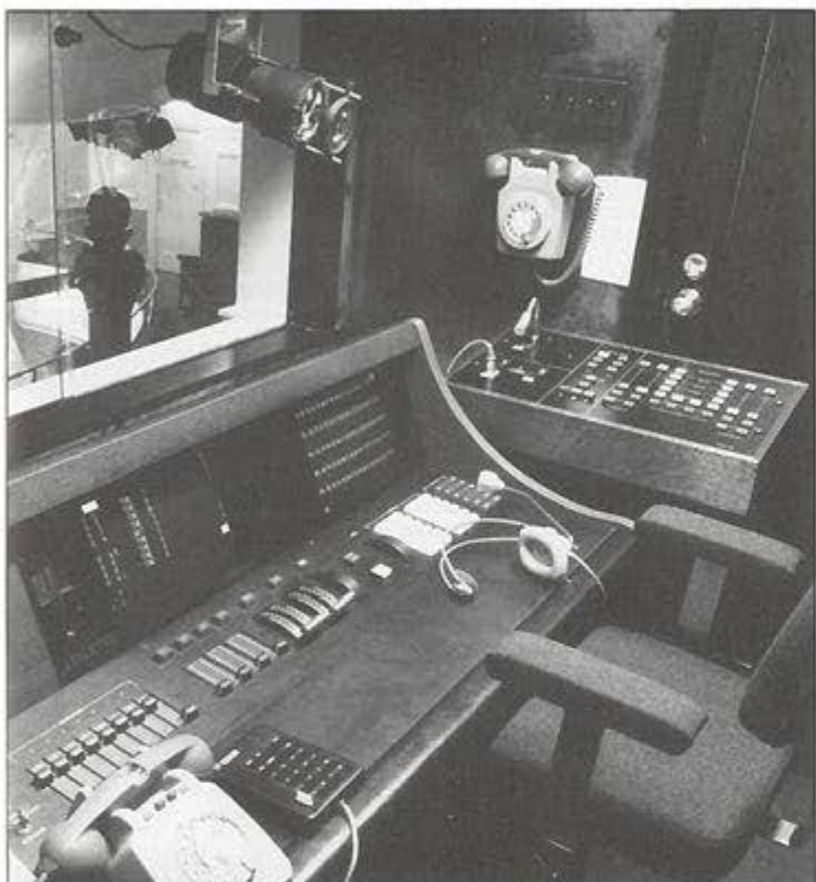
4 Revolve hydraulic motor speed range control. 5 Prompt corner combined facilities panel and communications rack. 6 Light Palette and Independents trolley.
