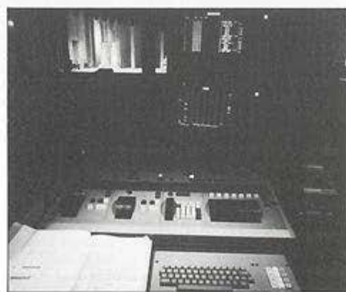
Lighting Control Room - operator's view on to the stage
