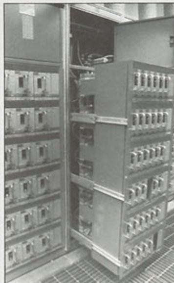
The dimmers are mounted in special "files" which slide out to allow access.
