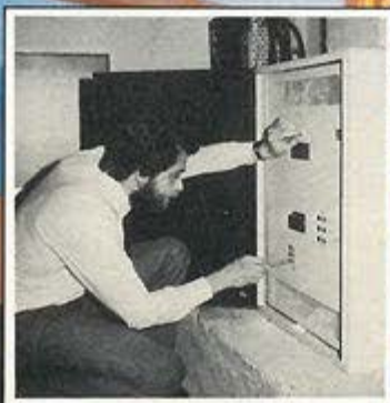
Paul Whitehead, Environ Technical Manager, sets the dimmers in the basement electrical plant room.
