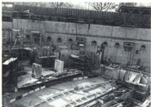
North end of excavation May '77 showing State auditorium floor slabs. Black rectangles 1/3 down concrete walls are ends of rock anchors.
