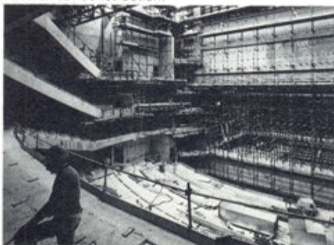
Interior of State Theatre looking towards stage, before roof construction.
