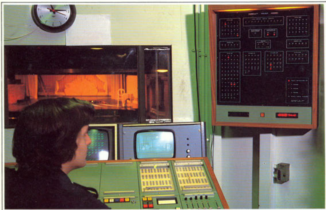
▲ View of the M.M.S. fault mimic and load limiter warning panel at the Albery Theatre. The fault mimic, a widely specified Strand option, indicates by a tell tale lamp if no current is passing in a circuit. Thus a blown lamp, fuse, or a dimmer fault or indeed any temporary disconnection can immediately be spotted by the operator.
