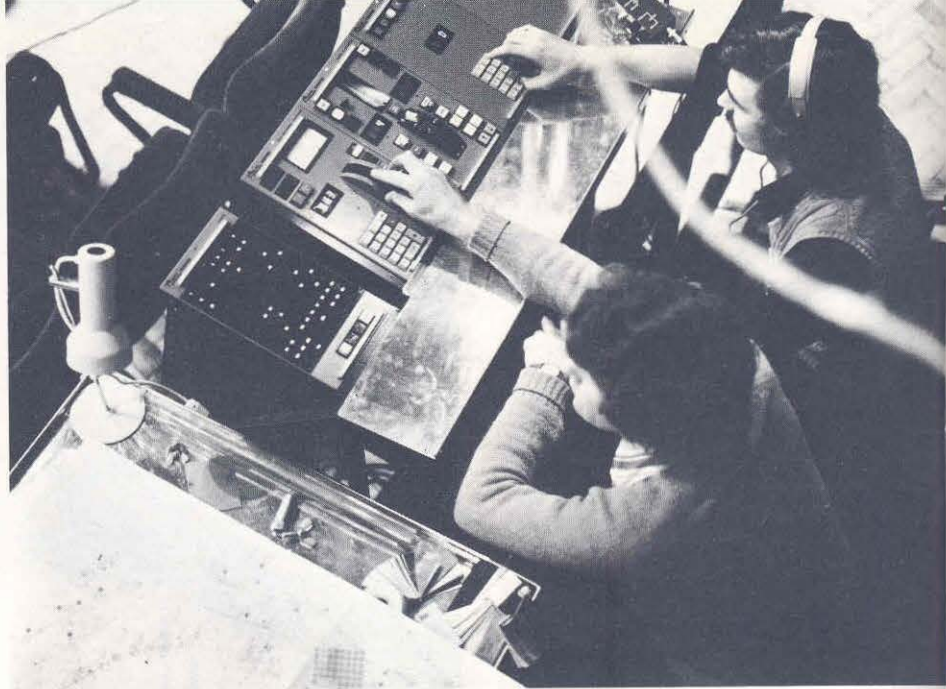
MMS lighting control removed to ground floor level for rehearsal
