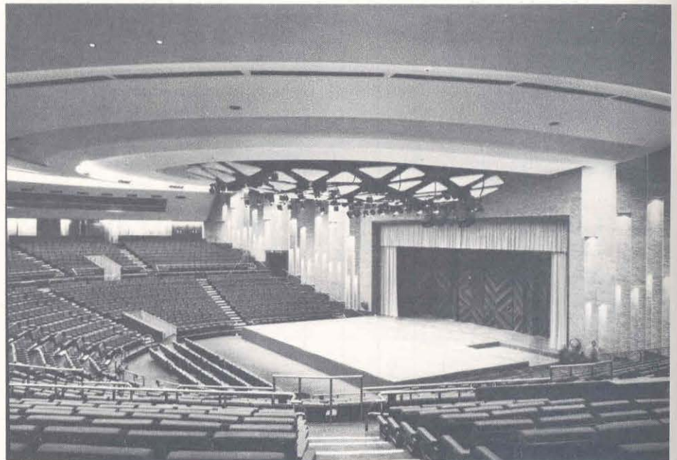
The main auditorium showing acoustic reflectors and proscenium walls.
