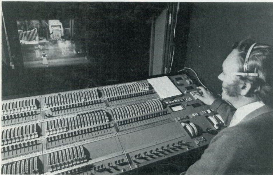
The Rank Strand System MSR control has been referred to in several of the preceding articles: That shown above is the 180 channel (150 fitted) MSR recently installed in Sadlers Wells Theatre, Rosebery Avenue, London.
