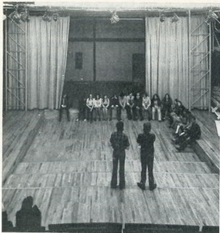
Drama studio, Loxford Comprehensive School, showing floor area removed to form a well.
