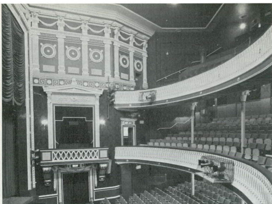
Liverpool Playhouse showing detailing of the 1911 auditorium carefully restored.
