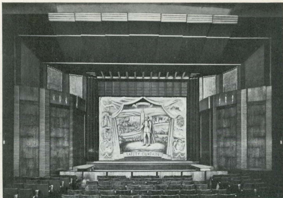
Stratford-upon-Avon. 1932 forestage two steps below main stage and with enclosed assembly areas either side.
