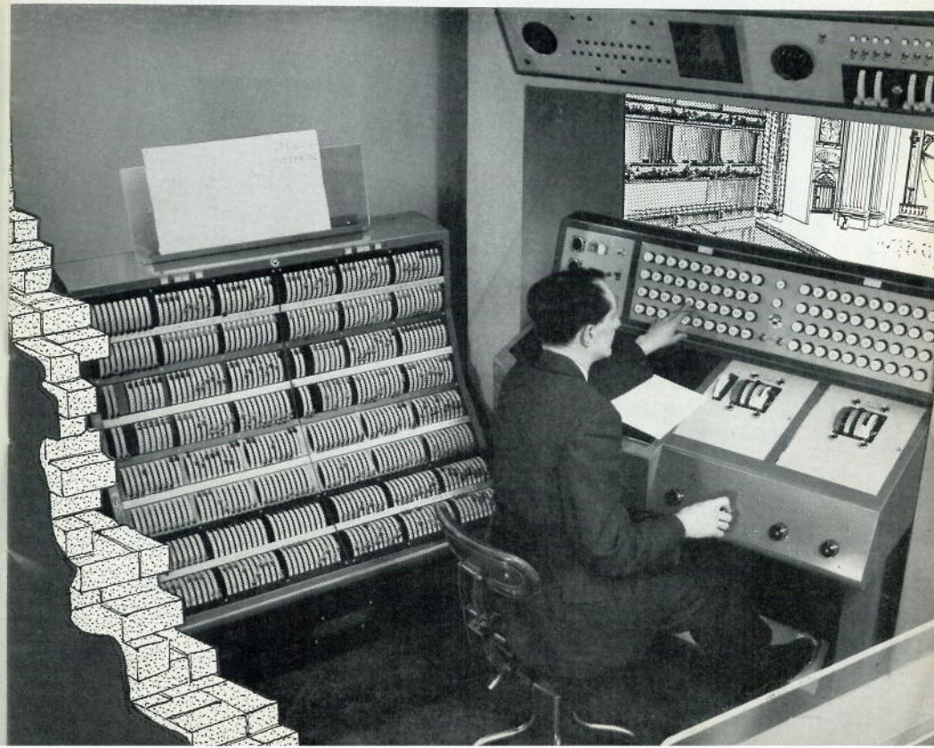
Lighting control at Covent Garden (faked at Gunnersbury works because of lack of space for camera shot). Controls over window are mainly for sound communication.
