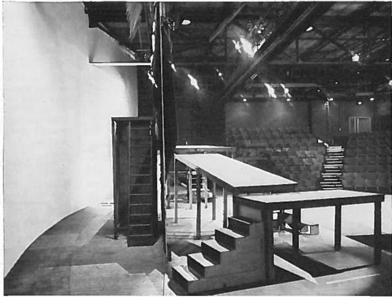
Fig. 3. View from off-stage O.P. side showing curved cyclorama on the left and scenic structures for "Brand" in foreground. Curtain track under lighting bridge is for house tabs when theatre is adapted to proscenium.
