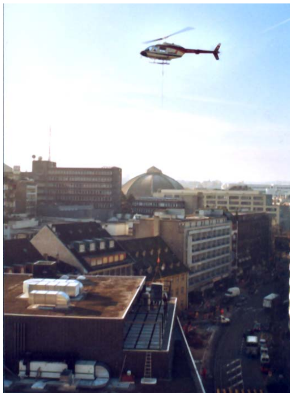
A helicopter lowers the dimmer racks into the theatre
