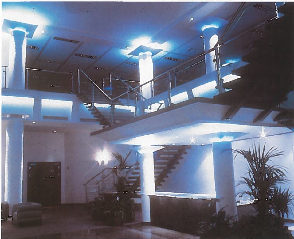
■ Whitebrook Park, Maidenhead: Metal halide downlights provide general lighting for the reception area to give an overall fresh, cool white light. Photos provided by Lighting Design Limited.
