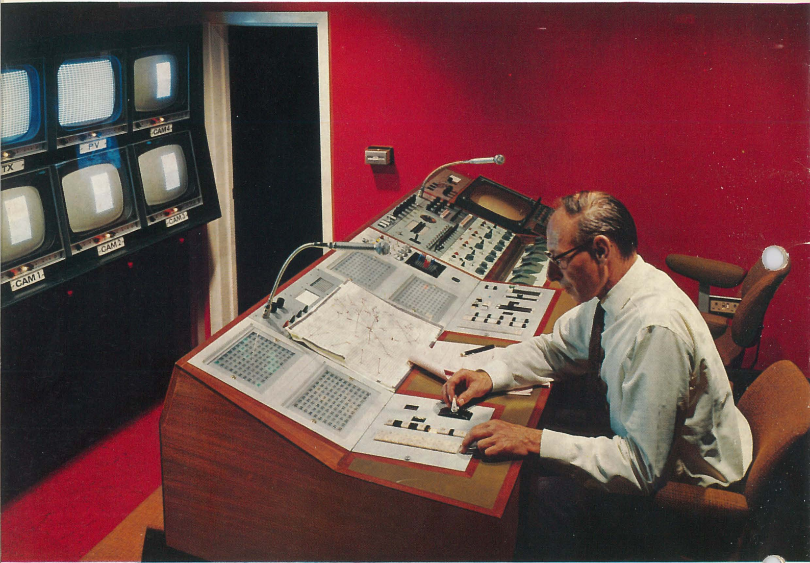
Q-File lighting control system in the Southampton studios of Southern Independent Television.
