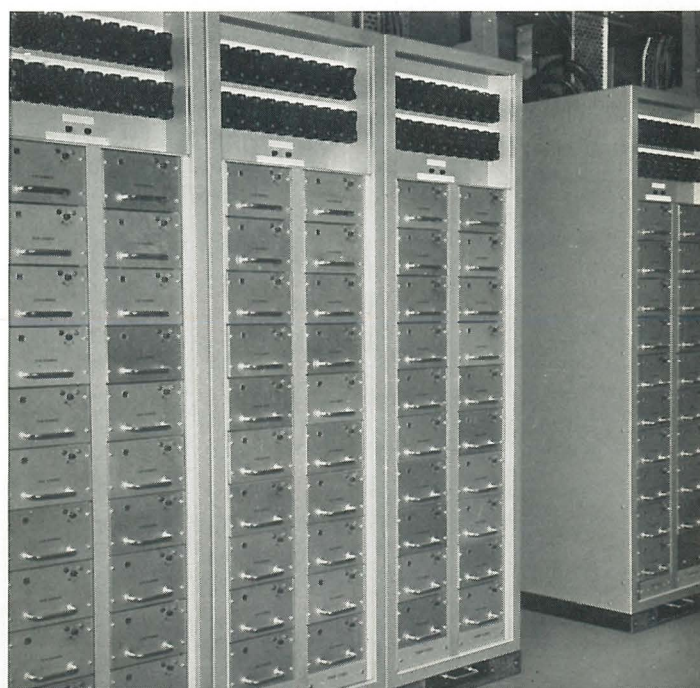
A typical Q-File dimmer room installation. Each rack provides 100 Kilowatts of dimmer capacity (5 Kilowatt dimmers are shown here).
