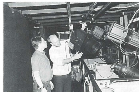
Howard Eaton (right) discusses his tracking follow-spots with production electrician Alistair Grant.
