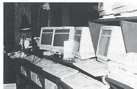
Control is provided by six Genesis computers with the operator's 'go' button just visible centre.
