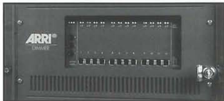
Diagnostic indicators and circuit breakers are clearly visible through the smoked glass door
