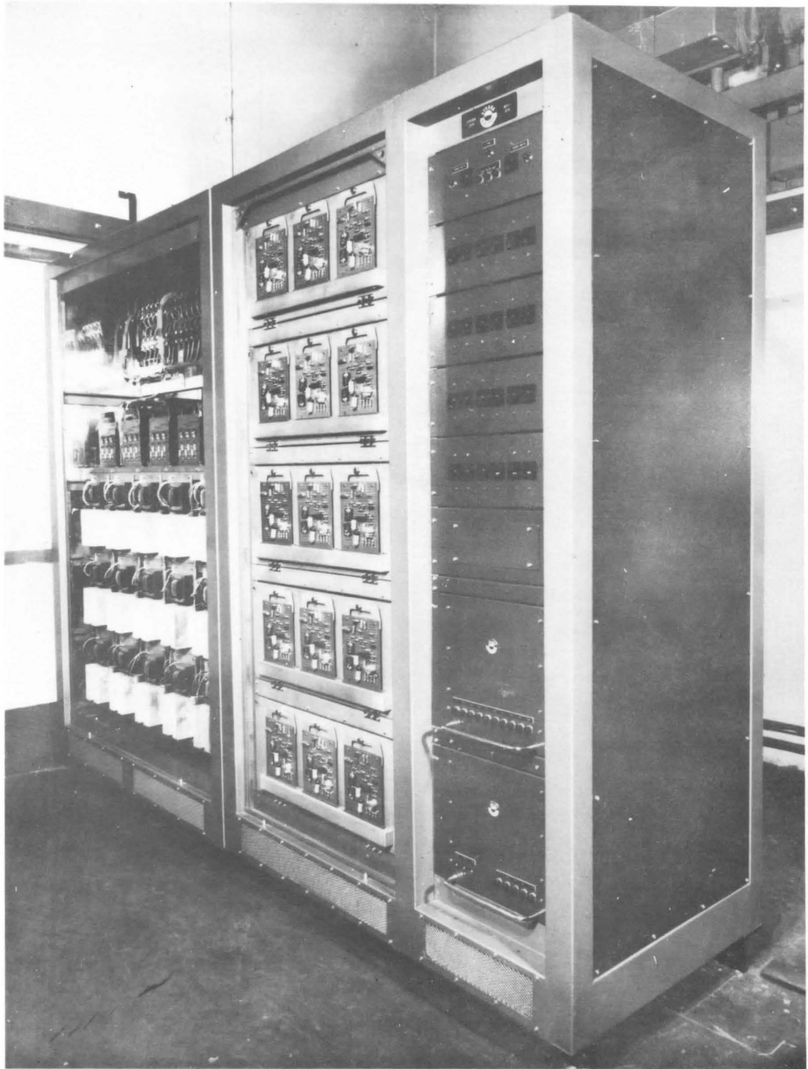
FIG. 1. System CRD self-contained rack with covers removed showing circuit breakers in foreground followed by 15 dimmer channels and clean-up unit at the far end. (A further 15 channels are housed at the rear).
