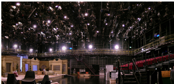
Figure 10. Tungsten house lighting in the TC4 studio
