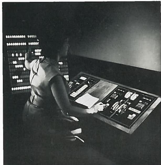
Rank Strand System DDM. Individual rocker tablet controls for 240 channels are on the wing. Dimmer memory controls and numerical selector to break sequence is on the left of the desk and the playback controls on the right.
