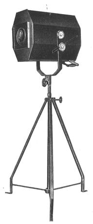
For the large stage, or where the general level of stage illumination is high, an arc lamp is essential, if satisfactory projection of optical effects is to be obtained. Although this lantern is primarily intended for use on the stage, it may be used with considerable success on front of house throws up to 100 ft., provided that provision is made for auxiliary support of the long lens tubes required. For throws over this, attention is drawn to the lanterns listed on pages 42 and 43.
