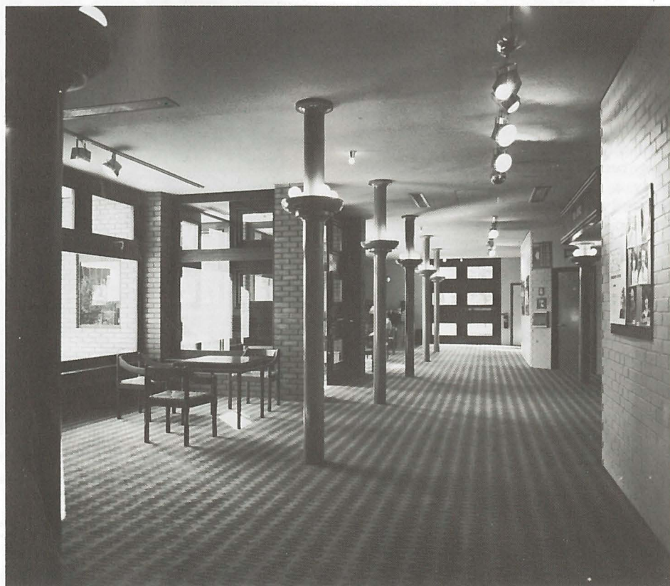
The columns are a feature of the design.
