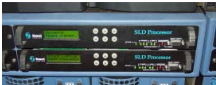
Each dimmer rack features dual dimmer processor electronics with Russian language displays
