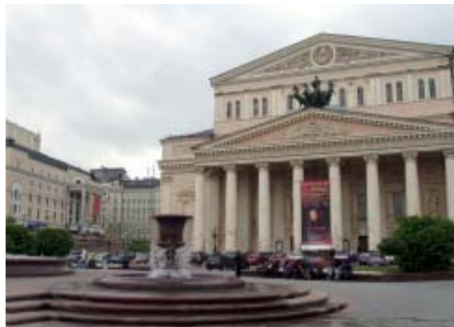
The main Bolshoi Theatre is shown here in the foreground with the Branch of the Bolshoi at the side
